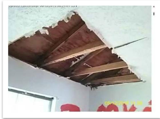
Removal of drywall and insulation.
