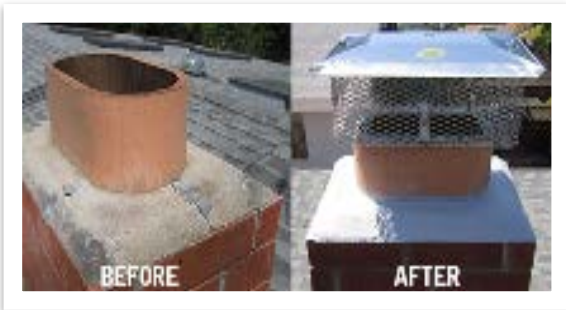
Example of one Chimney Cap Allowable used to cover a single flue.
