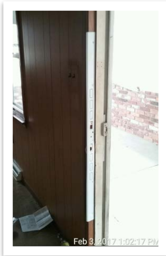
Photo shows door jamb protection product being installed.
